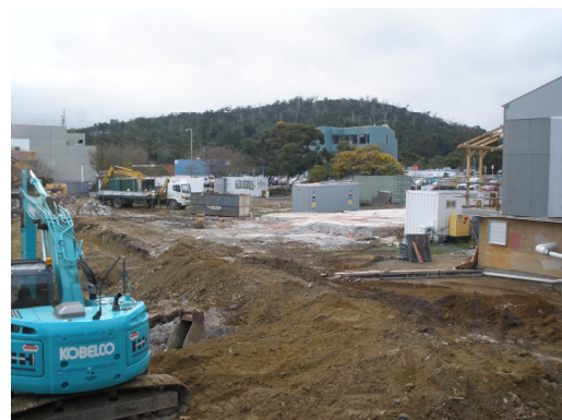
Stage 2 ICC Demolition Site
